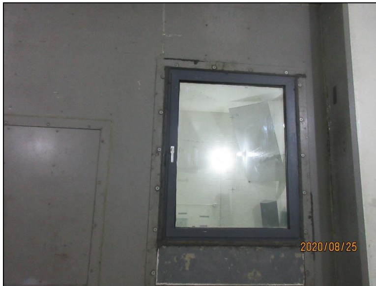
Photo No. 1 Receive Room View of Installed Test Specimen
